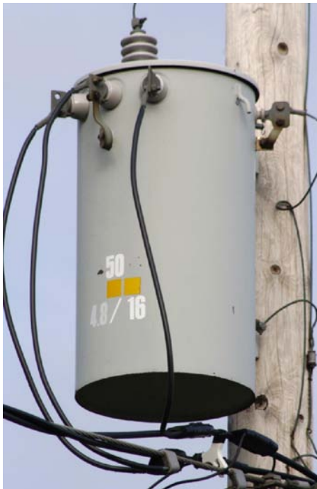
Figure 5 Single Phase Transformer 15
